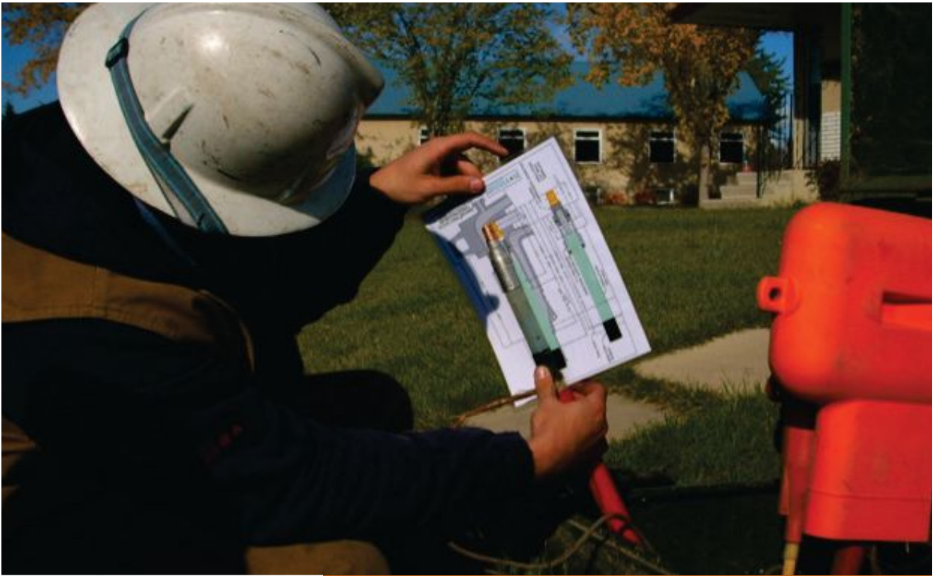
Figure 3. A craftsman in Alberta uses a template to make sure all of the cutbacks line up within appropriate tolerances. The component is shown in cut-away, so that the craftsman can visualize how his work fits within the internal mechanisms of the component.
