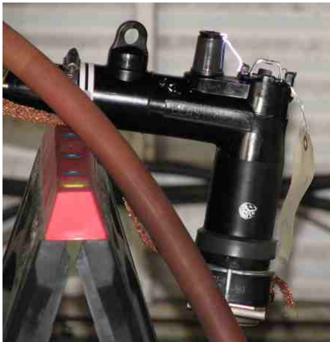
Figure 5: Flashover during another high voltage test.
