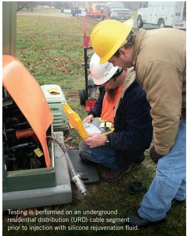
Testing is performed on an underground residential distribution (URD) cable segment prior to injection with silicone rejuvenation fluid.
