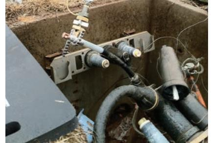
Sustained pressure rejuvenation (SPR) allows for faster completion of the injection process, making it an appealing choice especially for large cable rejuvenation projects.
