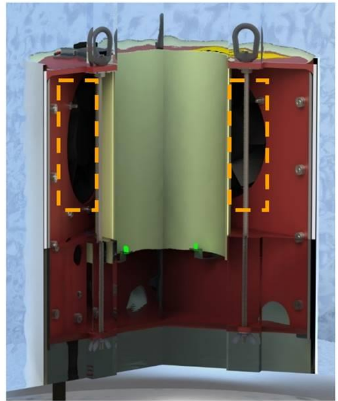
Fig. 3. Manhole event suppression system.
